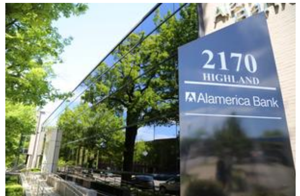
CW Holdings and Vulcan View Partners have purchased the former Alamerica Bank building in Five Points South.
